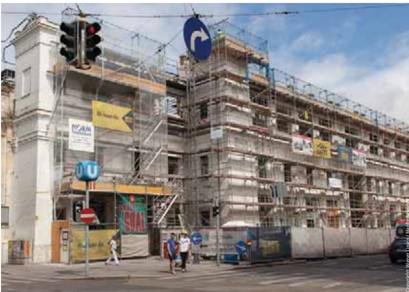
Exterior view of Alser Straße Station during renovation
