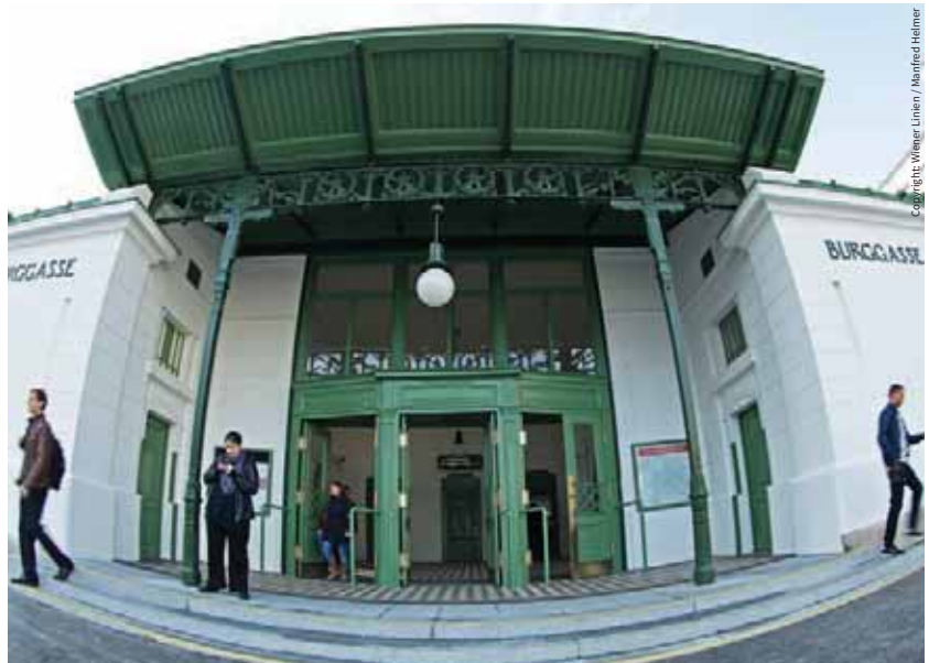
U6 Station Burggasse after renovation
