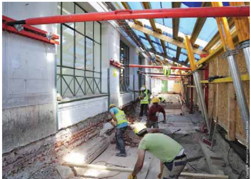
Platform demolition work at Alser Straße Station
